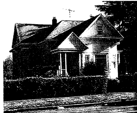
Homes in Portsmouth Neighborhood
